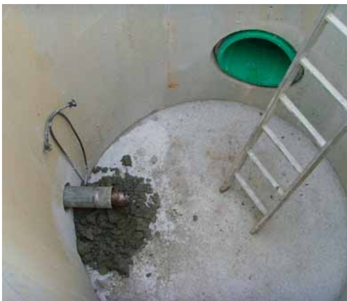
Arrival of the pilot bore in the target manhole.
