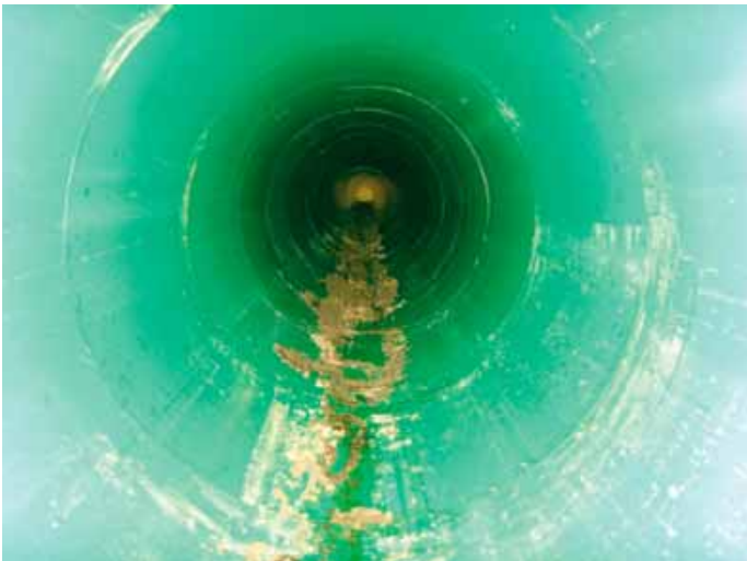
View of the installed product pipe made of PP-HM, system Schöngen
