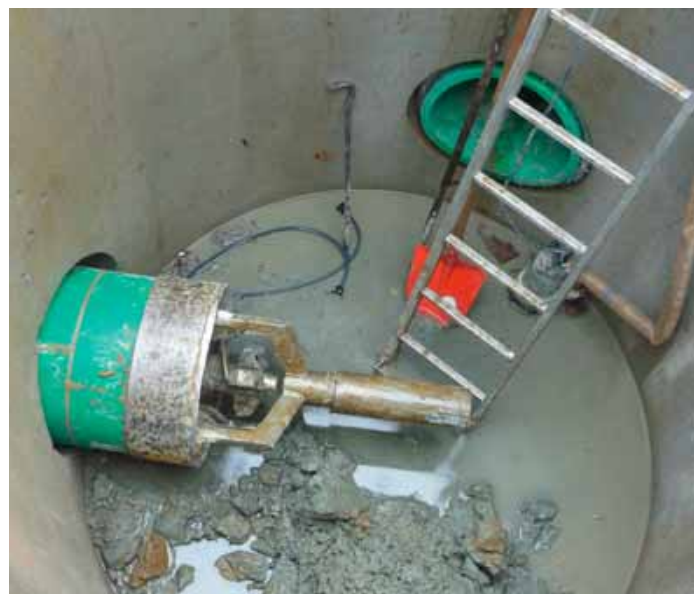
Arrival of the combined bore head in the target pit.
